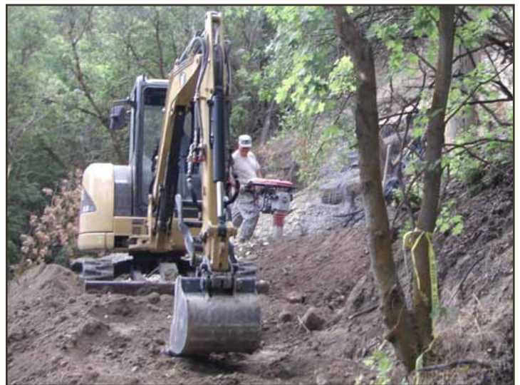
SGM David Hamilton compacting soil to augment stabilization of soil.
