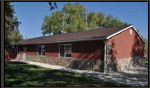
Building 6240 is classroom space that units reserve for training and is also used by VIPs for Governor's Day.
