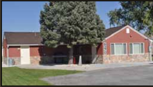
Building 6270 is the Sergeant Majors temporary quarters. Primary user for Building 6300 is Regional Training Institute billeting, but it is
